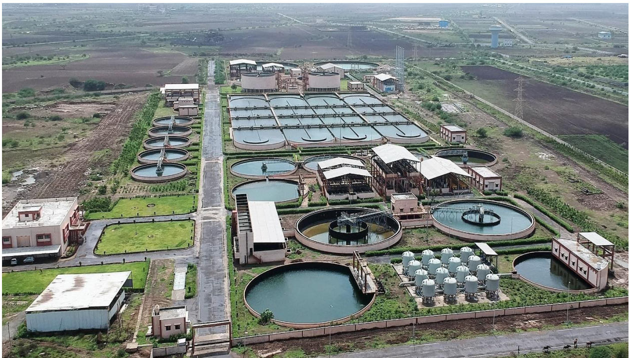
40 MLD COMMON EFFLUENT TREATMENT PLANT AT SAYKHA (IMAGE COURTESY – ENVIRO ASSOCIATE)
