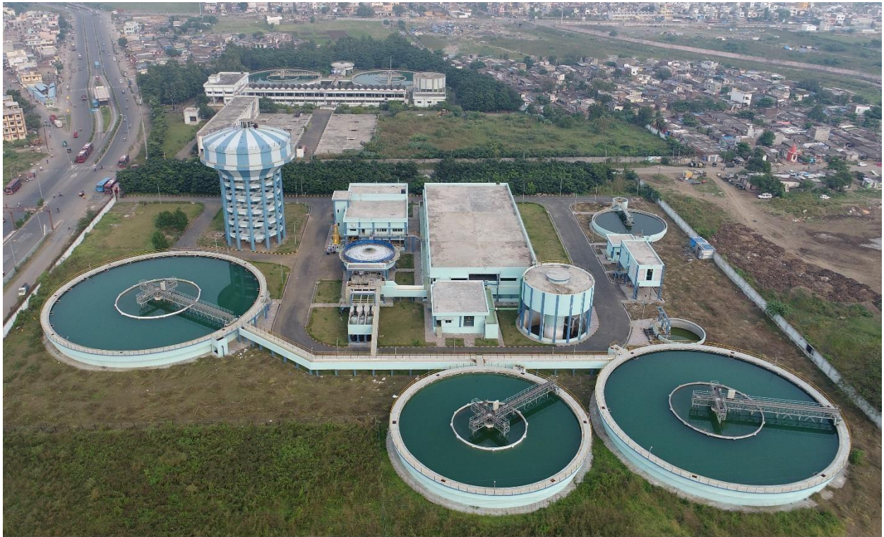
130 MLD WATER TREATMENT PLANT AT DINDOLI, SURAT (IMAGE COURTESY – ENVIRO ASSOCIATES)
